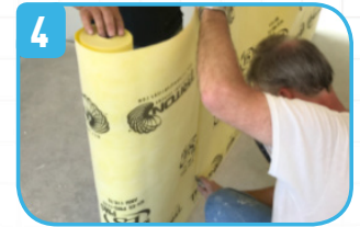
4 Precut WP™ Membrane to size including hole cuts for plumbing
