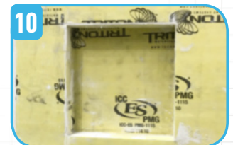
10 Niches and Bench Seats should also be covered with WP™ and treated with preformed corners.
