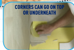
11 Apply WP™ Tape at membrane seams where 2" (50mm) overlap was not achieved. Use preformed WP™ corners at all inside and outside corner locations. Collars, corners, and seam tape can be applied underneath or on top of WP™ sheets.
