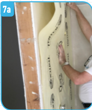
7a Align WP™ Membrane and embed into mortar.
