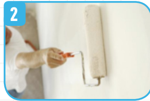
2 Drywall substrates need a coat of primer.
