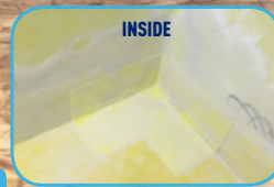
CORNERS CAN GO ON TOP OR UNDERNEATH
