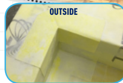
11 Apply WP™ Tape at membrane seams where 2" (50mm) overlap was not achieved. Use preformed WP™ corners at all inside and outside corner locations. Collars, corners, and seam tape can be applied underneath or on top of WP™ sheets.
