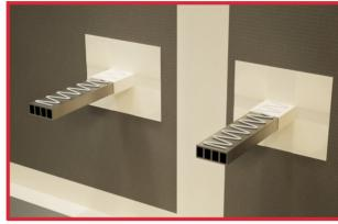
2. Install preferred backer board to manufacturer specifications. Then apply adhesive to both brackets.
